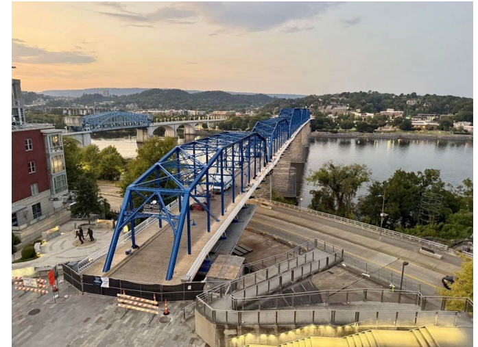
Walnut Street Bridge, Chattanooga.
